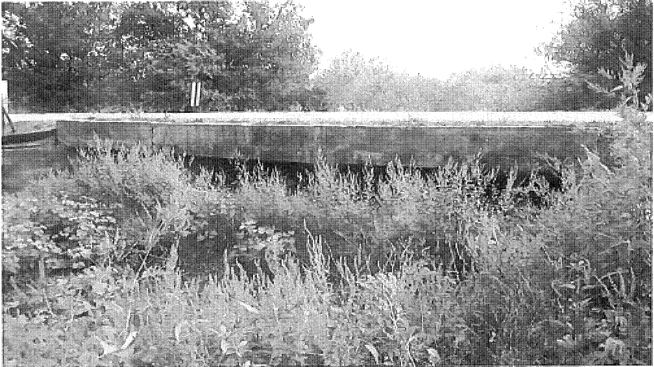
Figure 2: Culvert at Unnamed tributary of Elm Creek
